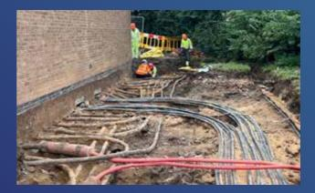
Extension pipes are used to reach depths which are not usually achievable when using a suction excavator. We have hundreds of metres of flexi extension pipe available for hire on request.
