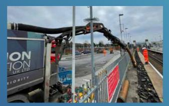
Our Triple Fan unit is identical to a 32T TRIDEM Suction Excavator, except that it has the added power of a third fan which provides supreme suction. When paired with our tracked Brokk system, the Triple Fan unit can excavate from a distance of up to 100m.
