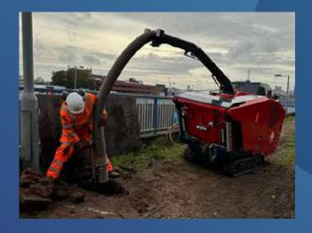
Our Tracked Vac is an all-terrain suction excavator which is perfect for hard to reach areas, fields, inner city developments, etc. This machine is perfect for lamp post columns, embankments, and other works requiring only small excavations. While the machine has its limitations due to its physical size and power output, it is surprisingly effective and you will be impressed with the productivity it achieves.
